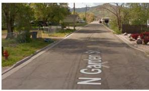
This section has curb and gutter throughout with about 26 feet of asphalt for the entire segment. With the gutter pan included the hard surface increases to 30 feet. There are 3 hydrants along this segment that are within code distances.
