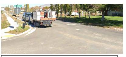
Segment is newly constructed. Access is adequate on South end. The asphalt widths are within the City Code standards except for the last 180 feet on the North end.
